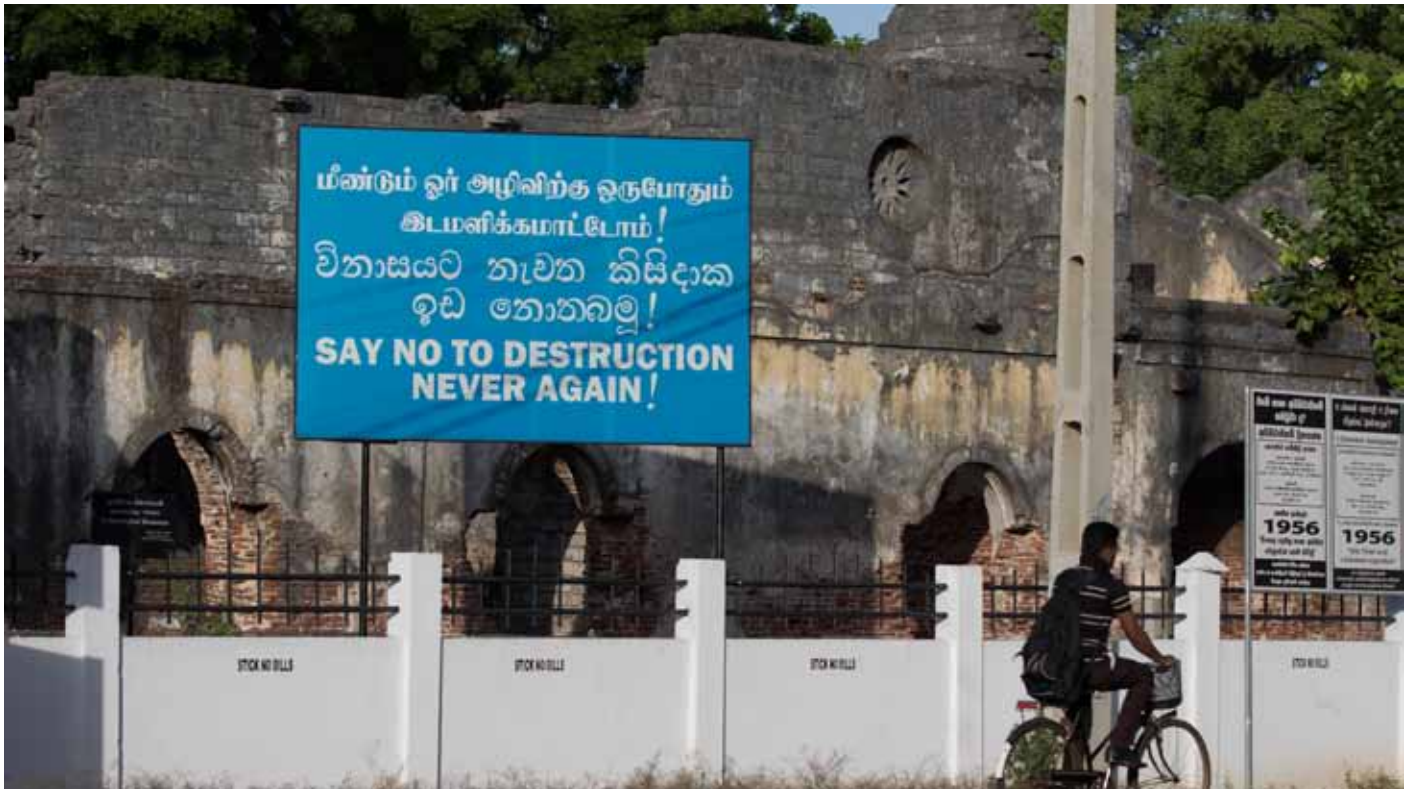
Cyclist riding past a building damaged by the war in Jaffna on 20 July 2015.
