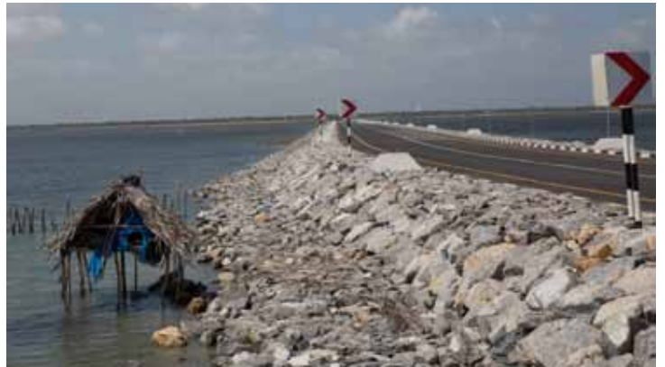
A newly built road across the Killai lagoon, North of Sri Lanka: brand new roads have not changed subsistence poverty levels.
